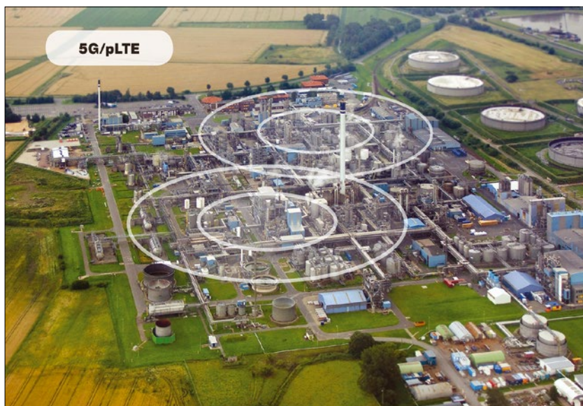
Figure 1: For the first time, 5G licenses enable private companies to set up their own campus networks.
